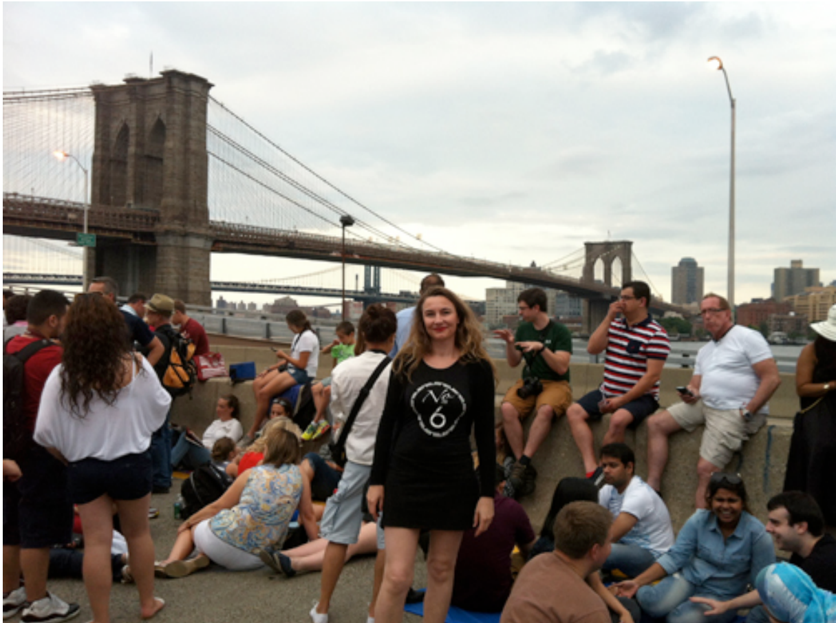
Kim Engelen [Bridges] Brooklyn Bridge, New York (USA) 2015
